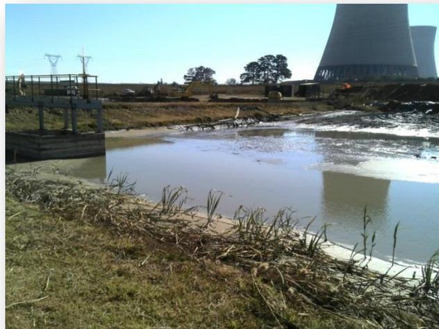
**Figure 7: Kendal PS Concrete lined Silt Trap with adjustable overflow weir**
