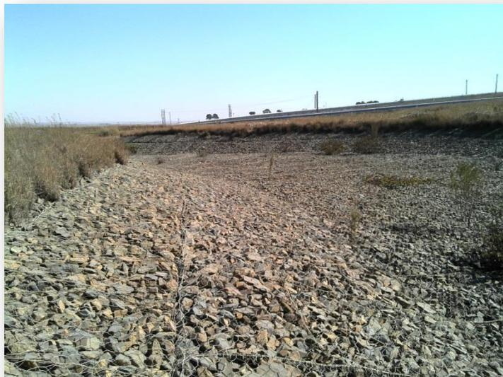
**Figure 9: Kendal PS Emergency Dirty Water Dam overflow channel**
